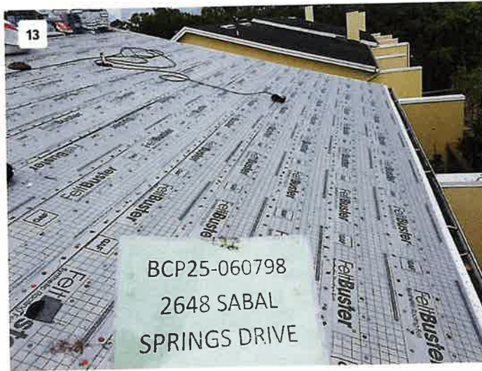
Project: 2648 Sabal Springs Dr unit 6 Date: Jul 7, 2025, 11:47 AM Creator: Lucio Roofer
