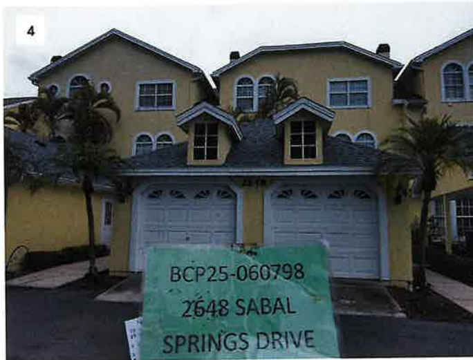
Project: 2648 Sabal Springs Dr unit 6 Date: Jul 15, 2025, 7:05 PM Creator: Lucio Roofer
